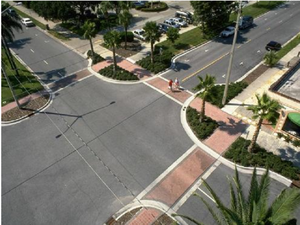
Figure 14.1 –Curb Extension (Neckdown)
