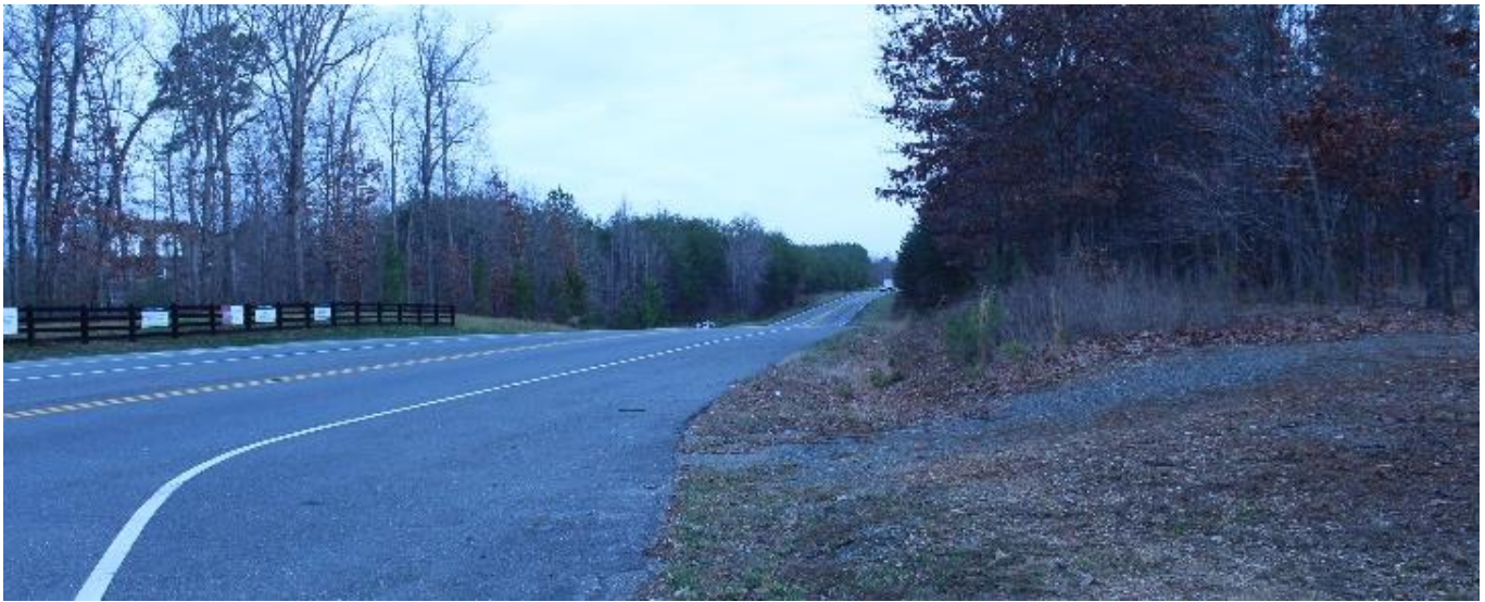
Figure 4 Westbound Approach on Spring Creek Parkway looking north along US 15 (Intersection #2)
