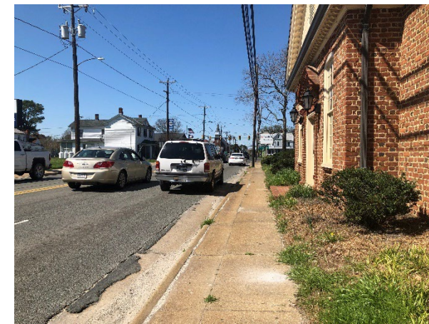
THE FIVE-FOOT WIDE SIDEWALK IS LOCATED IMMEDIATELY BEHIND THE BACK OF CURB WITH NO BUFFER. UTILITY POLES FREQUENTLY REDUCE THE THROUGH WIDTH. BUILDINGS ARE LOCATED WITHIN A FEW FEET OF THE BACK OF SIDEWALK.
