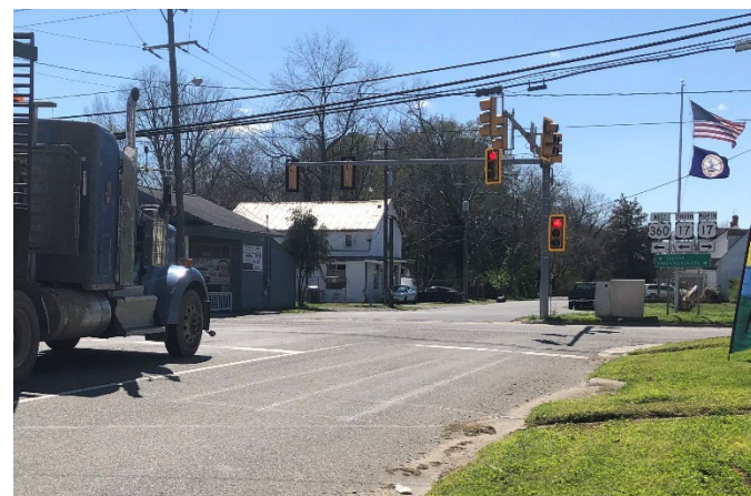
THE WESTBOUND APPROACH OF QUEEN STREET AT US 17 LACKS A DEDICATED LEFT TURN PHASE AND SIGNAGE INDICATING TURNING VEHICLES MUST YIELD TO ONCOMING EASTBOUND VEHICLES.
