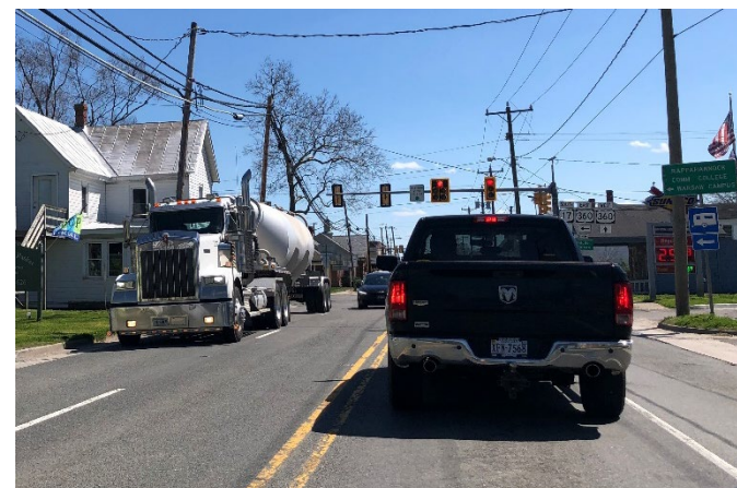
LANES ON US 17 BETWEEN MARSH STREET AND WRIGHT STREET ARE NINE-FOOT WIDE, PROVIDING LITTLE MARGIN FOR ERROR FOR VEHICLES CHANGING LANES. TRUCKS AND OTHER HEAVY VEHICLES COMPRISE 9 PERCENT OF DAILY TRAFFIC VOLUMES.
