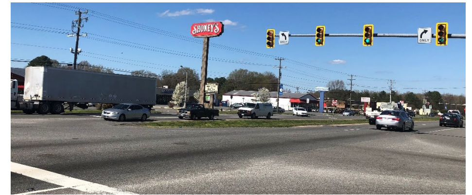
THE INTERSECTION OF BALL STREET AND US 17, LIKE THE OTHER INTERSECTIONS SOUTH OF HOSKINS CREEK, LACK PEDESTRIAN FACILITIES, INCLUDING CROSSWALKS AND PEDESTRIAN SIGNALS. A PEDESTRIAN CRASH OCCURRED AT THE BALL STREET INTERSECTION IN 2016.
