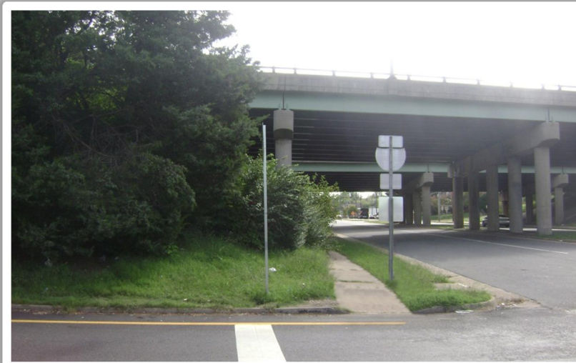
Photograph 2 – Looking East from I-195 Exit Ramp – Sight Distance Impacted by Vegetation
