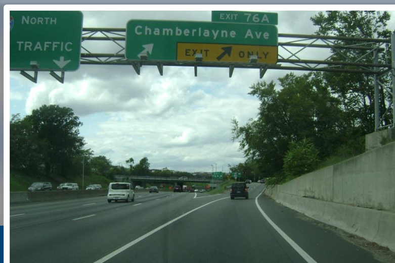
Photograph 2 – Off-Ramp to Chamberlayne Parkway - To be Removed
