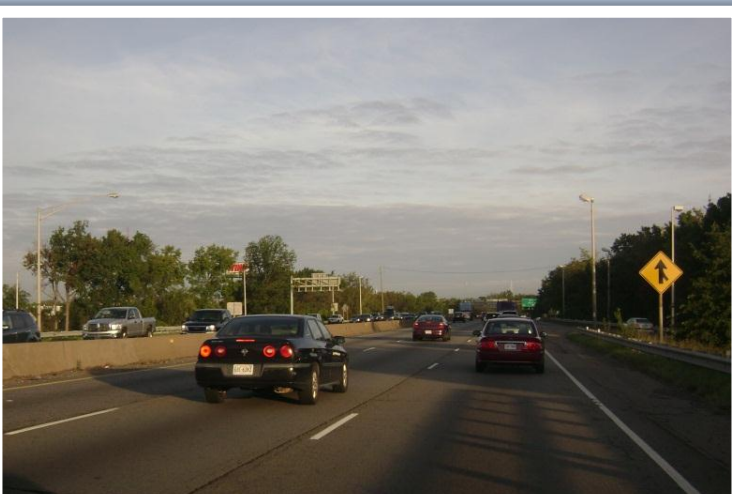
Photograph 2 – Northbound I-95/I-64 Weave Section between Bryan Park Interchange and Boulevard
