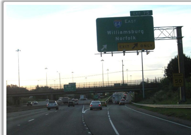
Photograph 1: SB I-95/EB I-64 East Interchange – High Mast Roadway Lighting
