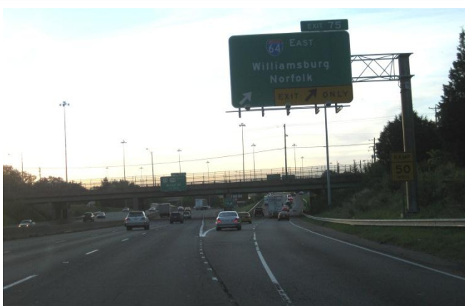
Photograph 1 – Interstate-to-Interstate Movement – Southbound I-94/I-64 Off-Ramp to Eastbound I-64
