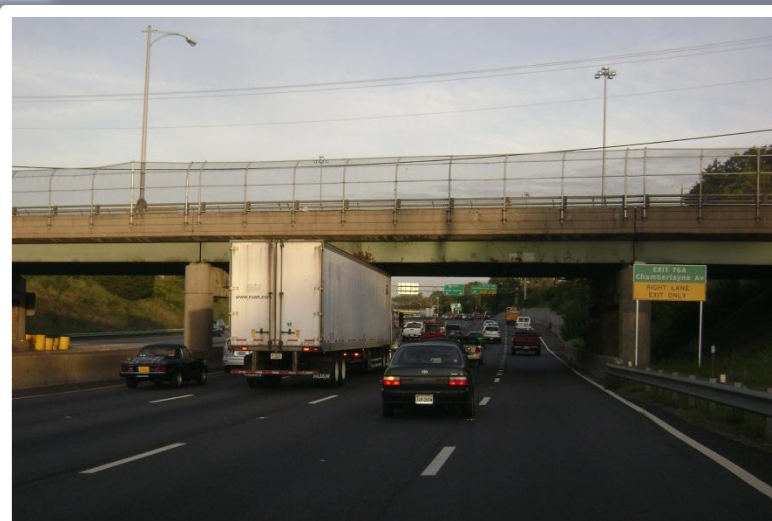
Photograph 1 – Northbound I-95/I-64 Weave Section between Westbound I-64 and Off-Ramp to Chamberlayne Parkway
