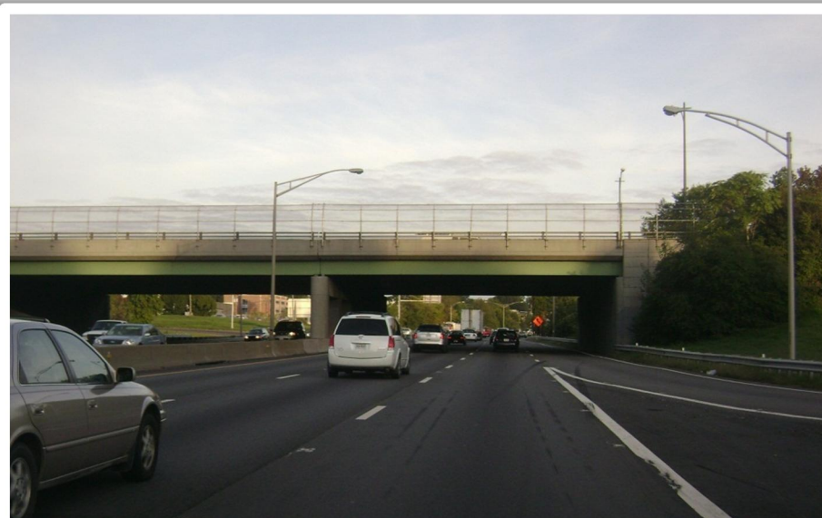
Photograph 1 - I-95/I-64 NB Approaching the Belvidere Street On-Ramp
