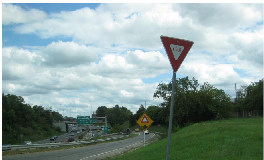
Photograph 2 – Looking East from Slip Ramp from Leigh Street
