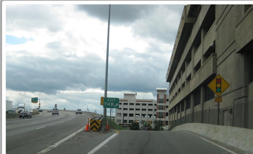
Photograph 1 – SB I-95 Exit Ramp to Franklin Street/15 th Street
